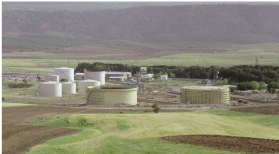
Khorram Abad Pump Station
